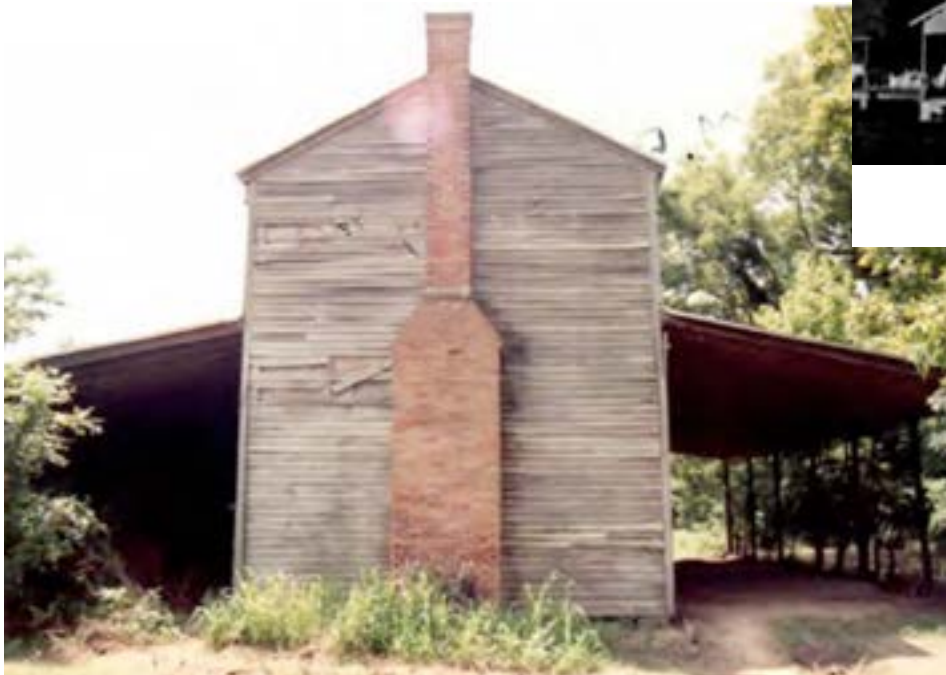
Figure 3: Tractor sheds attached to the house
