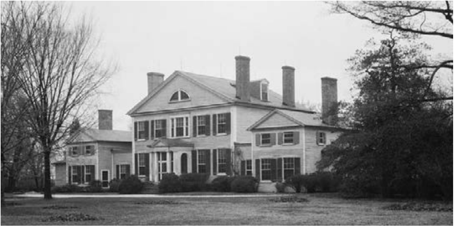
The Wye House Plantation mansion in Talbot County, Maryland. Since the property is still owned by descendants of the Lloyd family, no official tours offer access to the grounds or buildings on plantation where Douglass was a slave and where he revisited in 1881
